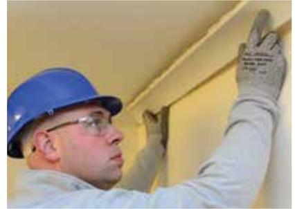
Gyproc Cornice Battens can be used to install Gyproc Cornice 135 over existing old cove profiles. Gyproc Cornice Strips can also be used to add extra steps prior to installing the Gyproc Cove.
