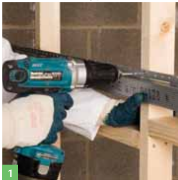
2 Resilient Bar fixed to one side
