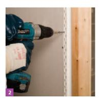
Insert the screw through the slot in the fin nearest to the centre line of the framing member, and fix using a slow speed screwdriver.
