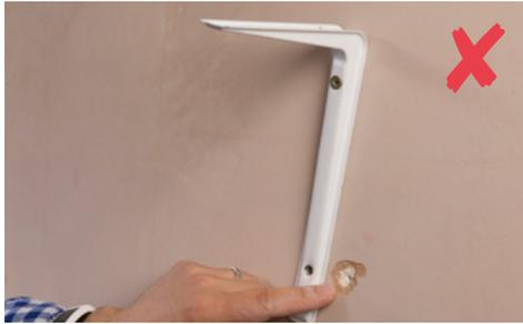
Incorrect fixing penetration through the board
