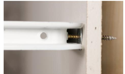
Sequence to show fixing pulling back through the plasterboard, effectively drilling a hole
