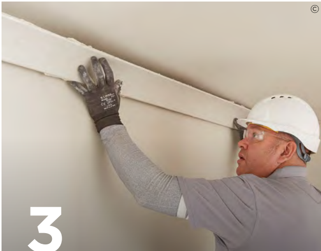
Nails are lightly applied to provide temporary support to the profile until the adhesive has set. Once set, temporary nails are removed and any excess adhesive is used to make good the mitres and any joints. After installation, surfaces are treated with Gyproc Drywall Primer prior to applying the decorative paint finish.
