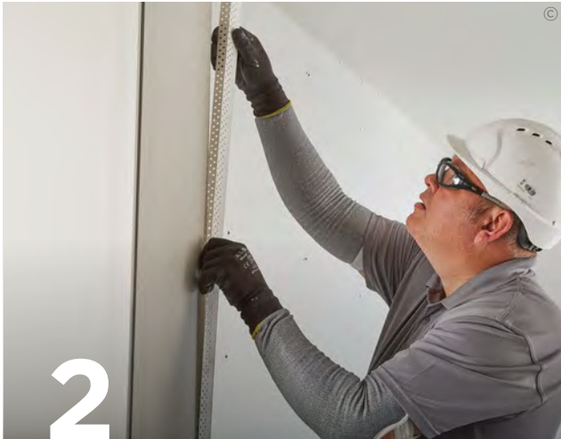
For external corners use the self-adhesive Gyproc AquaBead or Gyproc Corner Tape or Gyproc LevelLine which are bedded with a Gyproc setting compound.
