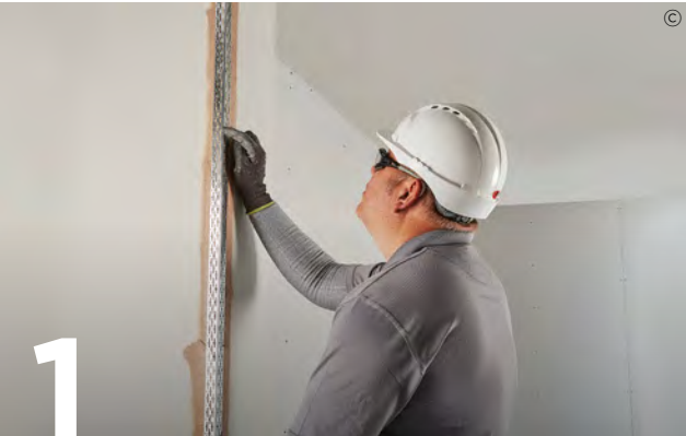
A Thistle Thin Coat Angle Bead is fixed to the plasterboard angle by embedding in dabs of finish plaster.
