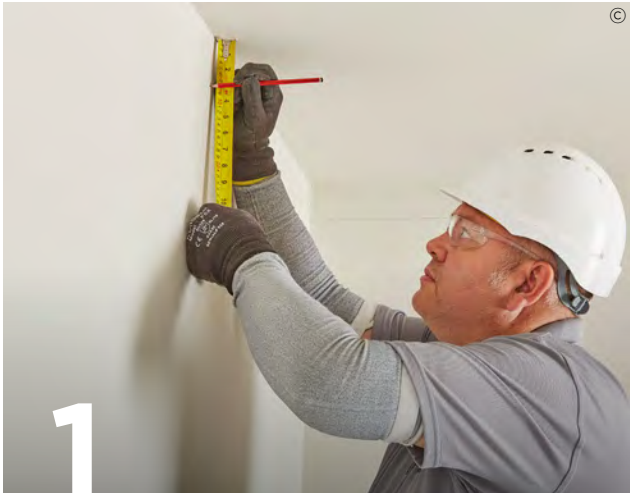
The positions of the cove or cornice are marked on to the wall and ceiling.
