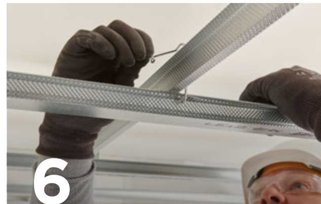
6 Alternatively, Gypframe MF9 Connecting Clips can be used in areas not prone to lifting.
