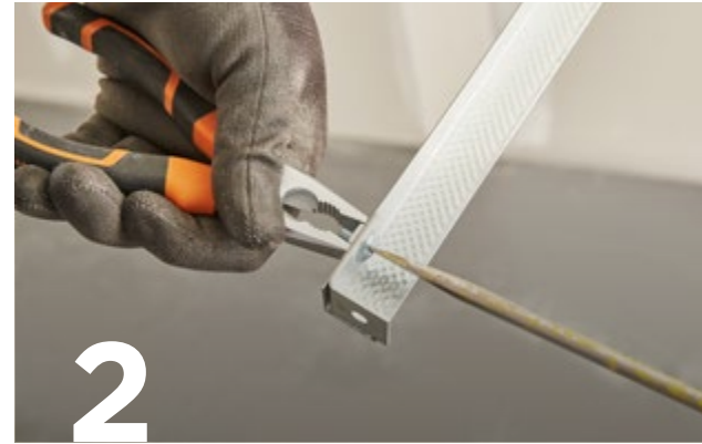
2 Form hangers by securing Gypframe FEA1 Steel Angle or Gypframe MF8 Strap Hanger to Gypframe MF12 Soffit Cleats with Gypframe MF11 Nuts and Bolts.
