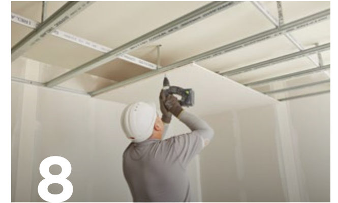
8 Use the appropriate fixing to fix Gyproc plasterboards, Glasroc specialist boards, Gyptone boards or Rigitone boards to the Gypframe MF5 Ceiling Sections and Gypframe MF6 Perimeter Channels.
