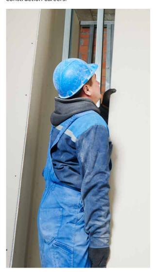
Construction involves moving, assembling and installing many types of potentially hazardous items or loads to create a finished building. The heaviest items always require mechanical handling, for example craning of preformed floor slabs, but many other types of handling such as plasterboard handling fall within a weight range where either mechanical or manual handling, or a combination of the two is possible.
