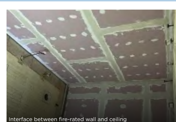
Interface between fire-rated wall and ceiling
