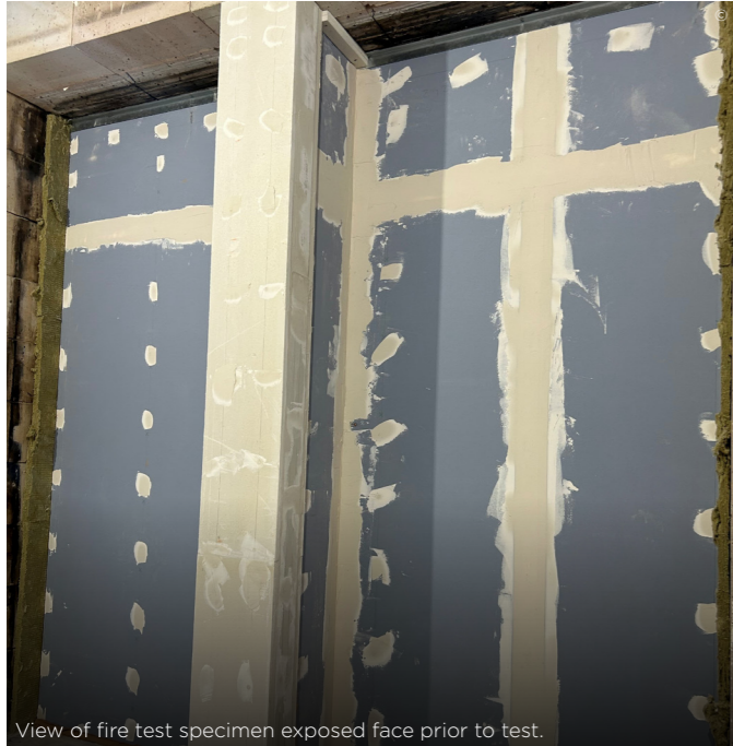
View of fire test specimen exposed face prior to test.
