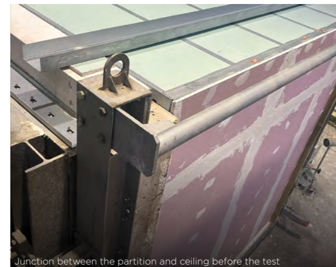
Junction between the partition and ceiling before the test
