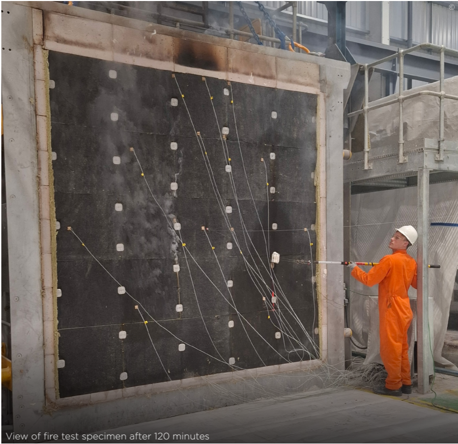
View of fire test specimen after 120 minutes
