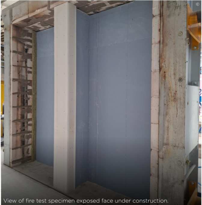
View of fire test specimen exposed face under construction.
