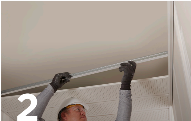
Cut CasoLine Main Tee sections to suit the width of the corridor. Main tee sections are then fitted into the CasoLine perimeter onto the upper recessed flange.
