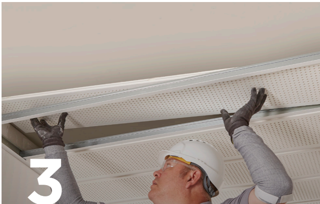
Cut Gyptone Planks to fit on the lower flange of the chosen perimeter component.
