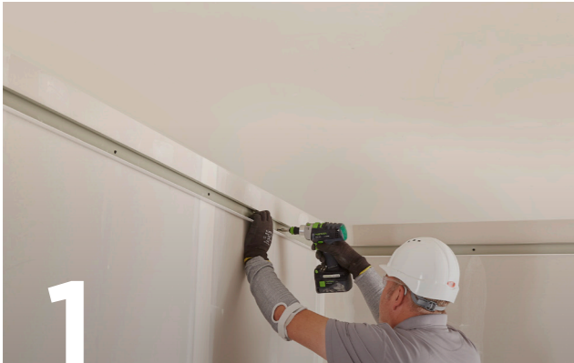
Measure and mark the required ceiling height. Fix the appropriate CasoLine Quick-Lock Corridor System component around the perimeter of the ceiling area.
