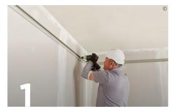
Place the CasoLine Quick-Lock Grid Wall Angle against the wall and ensure it's level, fix with suitable fixings at maximum 300mm centres.
