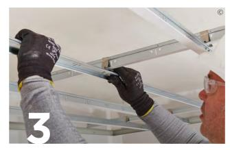
When installing D2 tiles place Cross Lock connectors a centre distance of 600mm on the CasoLine Quick-Lock Main Tee 24/38 (maximum 600mm from the wall).
