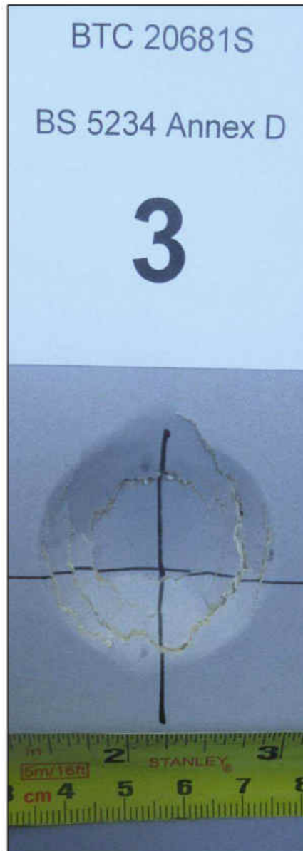
Photograph 1. Example of damage caused by the Annex D – Determination of resistance to perforation by small hard body impact
