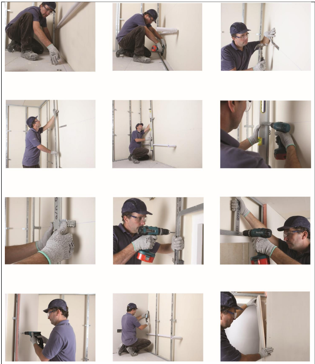
Figure 3 GypLyner SINGLE installation details
