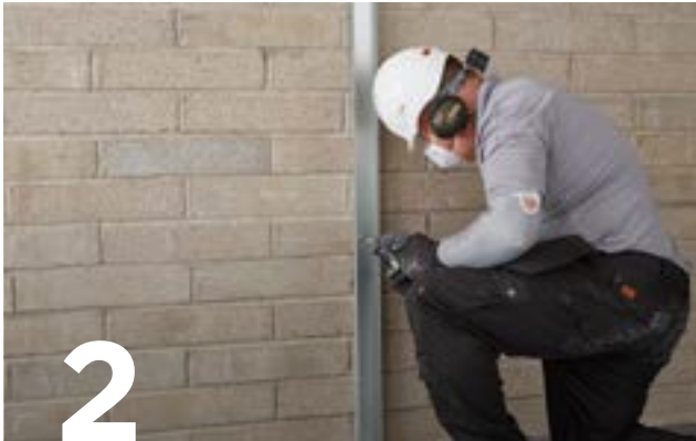
Suitably fix Gypframe Starter Channels to vertical abutments.
