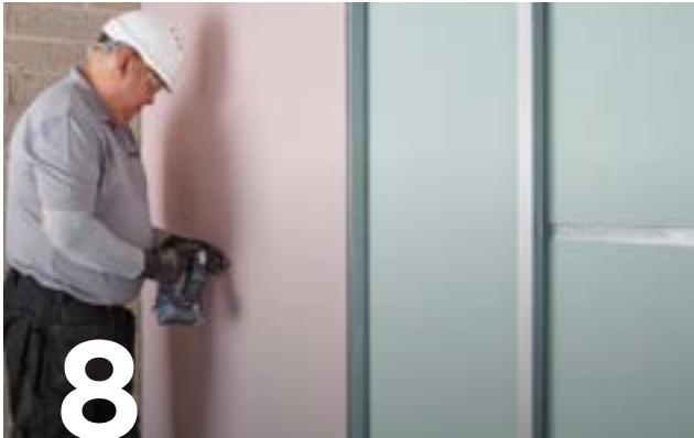
Gyproc plasterboard or Glasroc F FireCase are then fixed to the Gypframe framework with British Gypsum Drywall Screws to metal framing less than 0.8mm thick ('I' Studs less than 0.6mm thick) or British Gypsum Jack-Point Screws to metal framing 0.8mm thick and greater ('I' studs 0.6mm thick and greater).
