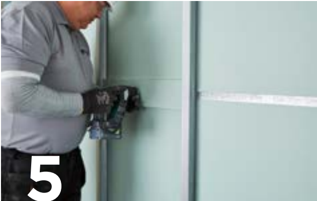
Fire stop horizontal board joints using Gypframe GA3 Angle and strips of Gyproc CoreBoard from the non-shaft side.
