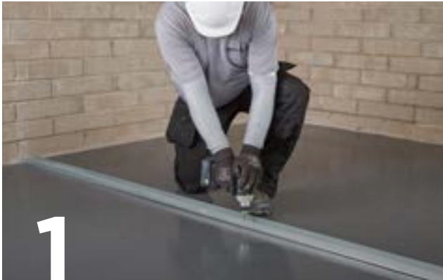
Suitably fix the appropriate Gypframe floor and ceiling channels to the perimeter at the required centres. Important note - for channels 72mm and below a single row of fixings are used. For anything above 72mm two rows of 600mm fixings staggered by 300mm are used. NB for def heads see suitable details
