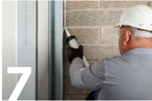
7 Use Gyproc Sealant to seal the perimeter.
