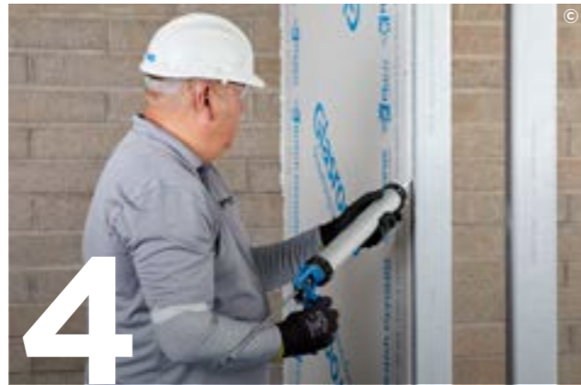
4 Run a continuous 6mm bead of Glasroc X Sealant along the installed Glasroc X Sheathing Boards exposed edges, which will have other boards abutting against it
