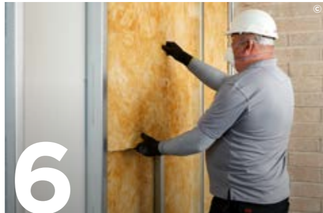
6 Add appropriate Isover insulation within the cavity.
