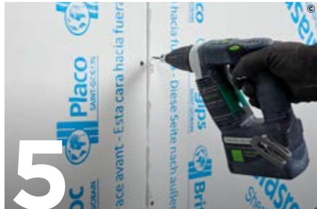
5 Abut subsequent sheets of Glasroc X Sheathing Board up to the previous one ensuring the sealant "mushrooms" out onto the face of the board, fully sealing the joint.
