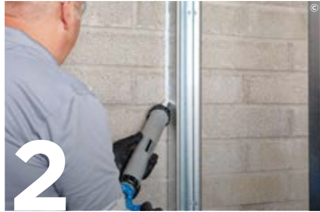
2 Before offering any boards into position a continuous 6mm bead of Glasroc X Sealant is needed along the vertical edge of the surface that the first sheet of Glasroc X Sheathing Board will abut.
