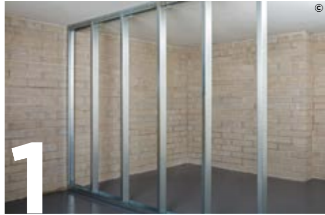
1 Completed Steel Framing System (SFS) framework ready to receive the Glasroc X Sheathing Board.
