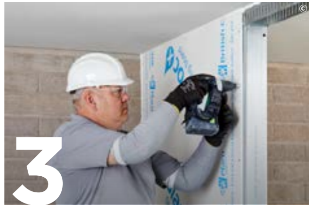
3 Use Glasroc X Screws 25mm to fix Glasroc X Sheathing Board to the SFS framework.
