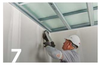
Use Gyproc Sealant to seal the perimeter of the frame.
