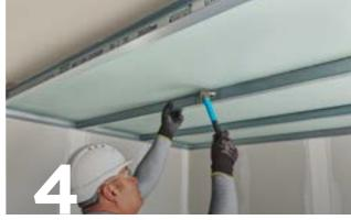
Use appropriate Gypframe Retaining Channels to hold boards in place.
