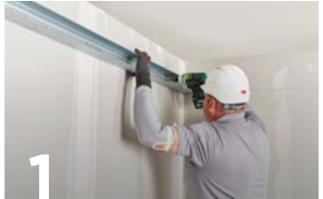
Suitably fix the appropriate Gypframe floor and ceiling channels to the perimeter at the required centres.
