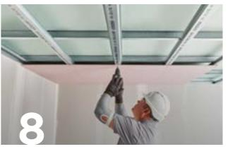
Gyproc plasterboards are then fixed to the Gypframe framework with British Gypsum Drywall Screws to metal framing less than 0.8mm thick ('I' Studs less than 0.6mm thick) or British Gypsum Jack-Point Screws to metal framing 0.8mm thick and greater ('I' studs 0.6mm thick and greater).
