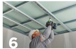
Run and fix Gypframe MF5 Ceiling Sections perpendicular to 'I' Studs using appropriate fixings.
