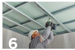
Run and fix Gypframe MF5 Ceiling Sections perpendicular to 'I' Studs using appropriate fixings.
