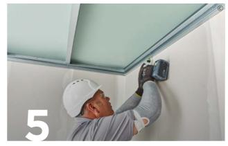
Fix the Gypframe MF6 Perimeter Channel directly to the starter channel and floor and ceiling channels using appropriate fixings.
