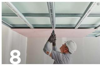
Gyproc plasterboards are then fixed to the Gypframe framework with British Gypsum Drywall Screws to metal framing less than 0.8mm thick ('I' Studs less than 0.6mm thick) or British Gypsum Jack-Point Screws to metal framing 0.8mm thick and greater ('I' studs 0.6mm thick and greater).
