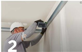
Position the appropriate Gypframe Starter Channels within the chosen floor and ceiling channel. Suitably fix to the perimeter at the required centres.
