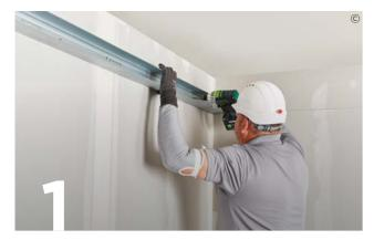
Suitably fix the appropriate Gypframe floor and ceiling channels to the perimeter at the required centres.
