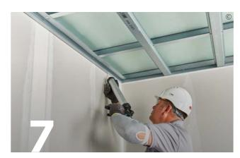
Use Gyproc Sealant to seal the perimeter of the frame.
