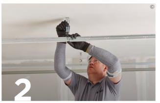
Place CasoLine Quick-Lock Grid Hangers for the CasoLine Quick-Lock Main Tee 24/38 at 1200mm rows. Squeeze the hook of the hanger together with a pair of pliers. The hangers should be adjusted, so the CasoLine Quick-Lock Main Tee 24/38 is elevated 44mm above the wall angle.
