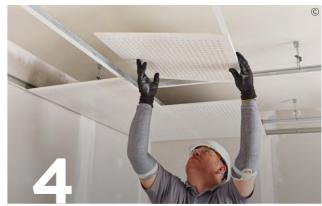
When installing the Gyptone edge D2, lift the E edge side of the tile, the E edge up above the cross profile. Then slide the opposite side of the tile, the D2 edge, into the opposite cross profile. When the tile is mounted in the grid system, it can be slide into place.
