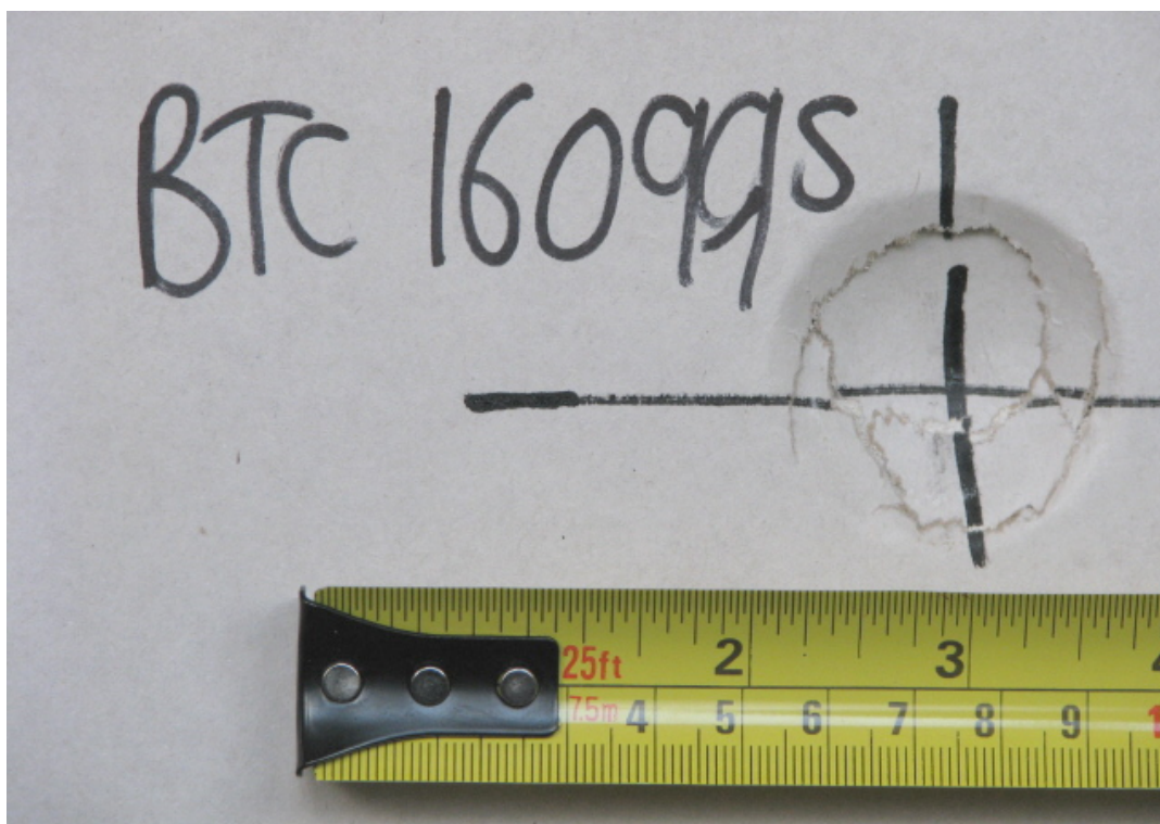
Photograph 2. Example of damage caused by the Annex D test for BTC 16099S.
