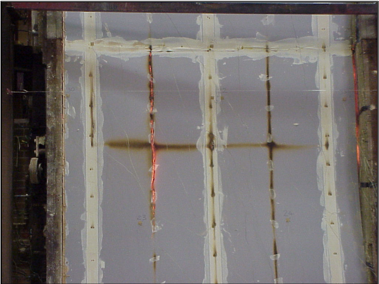
Photograph 4. Position of integrity failure at 118 minutes.
