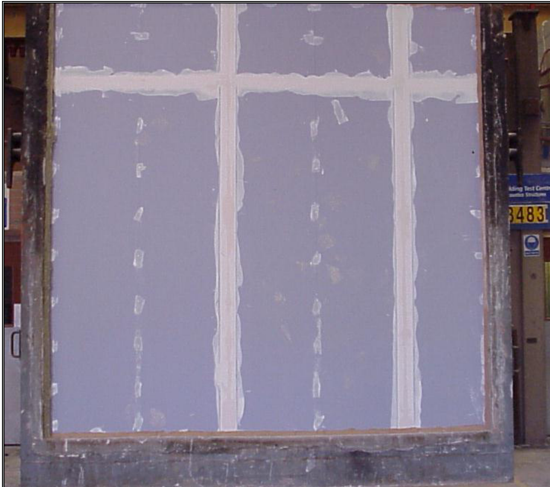
Photograph 1. View of the exposed face prior to test.
