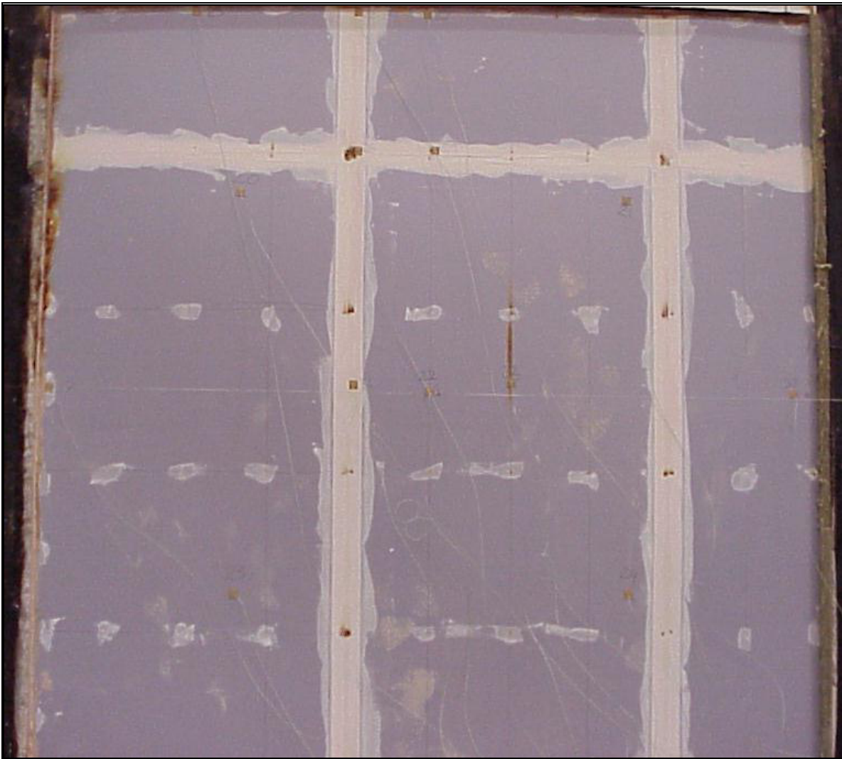
Photograph 3. View of the unexposed face at 102 minutes (after insulation failure).
