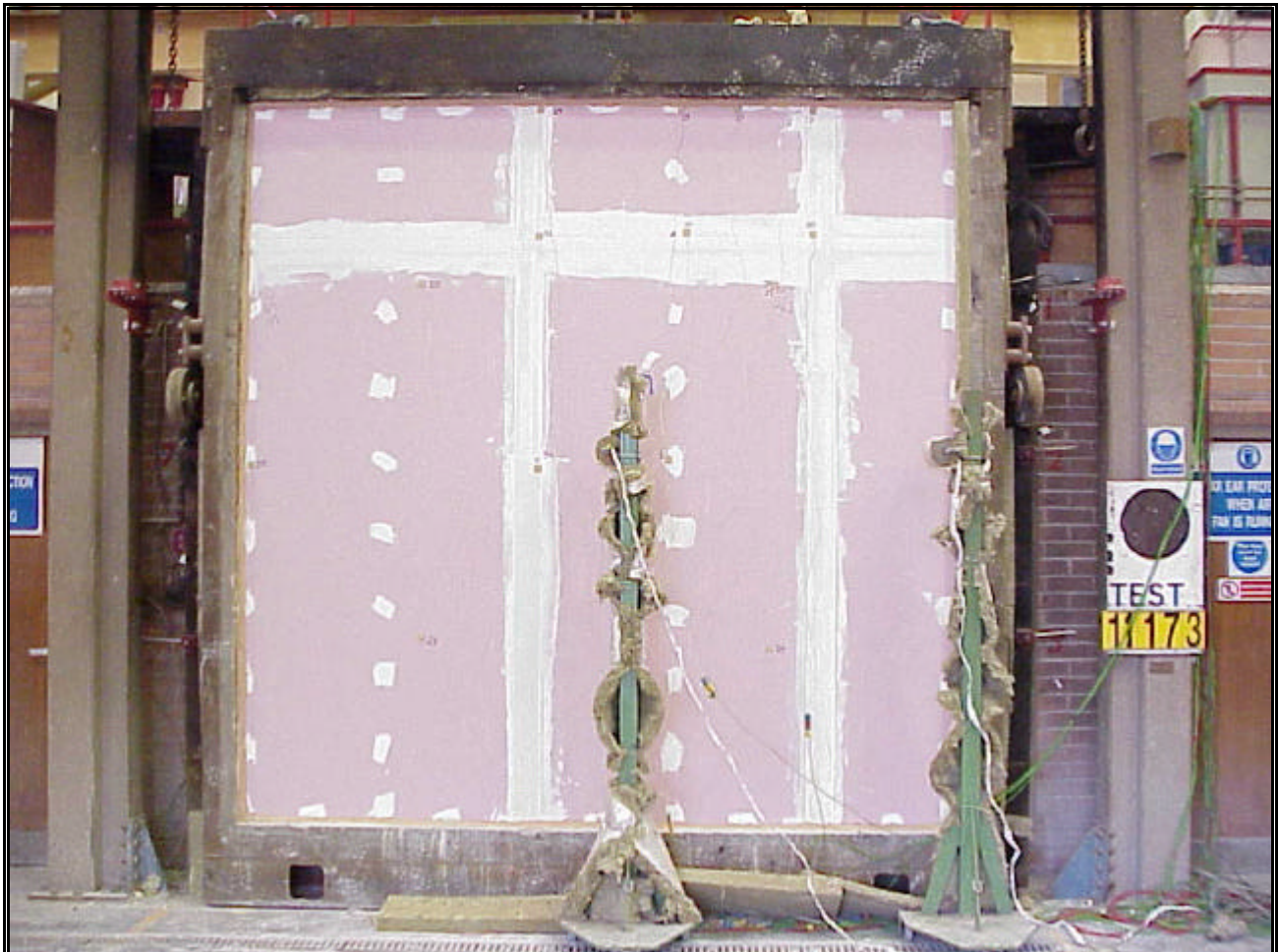
Photo 2. Unexposed face prior to test
