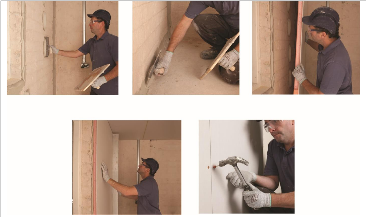
Figure 3 DriLyner DAB (Adhesive Variant) installation details
