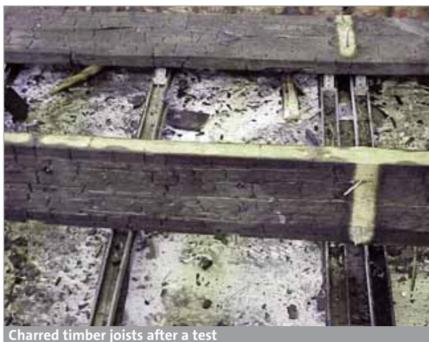
Charred timber joists after a test
