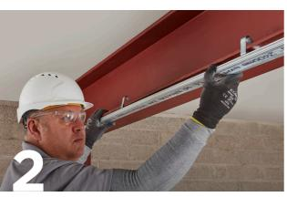
Locate Gypframe GL1 Lining Channels over the clips to form the steel framework.
