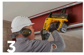
For two or three-sided beams or columns, use appropriate fixings to secure Gypframe GA2 Steel Angles to both sides of the wall / soffit flange.
