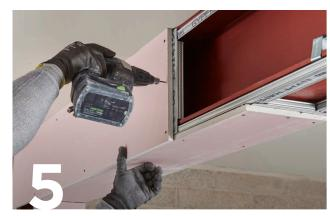
For single layer beam encasements board-end joints are backed using vertical noggings formed from an appropriate Gypframe component: Gypframe GL1 Lining Channel, Gypframe GFS1 Fixing Strap or Gypframe GFT1 Fixing 'T'.
